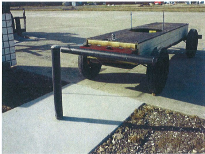
Figure 6 RB-2 Bollard Prior to Testing
